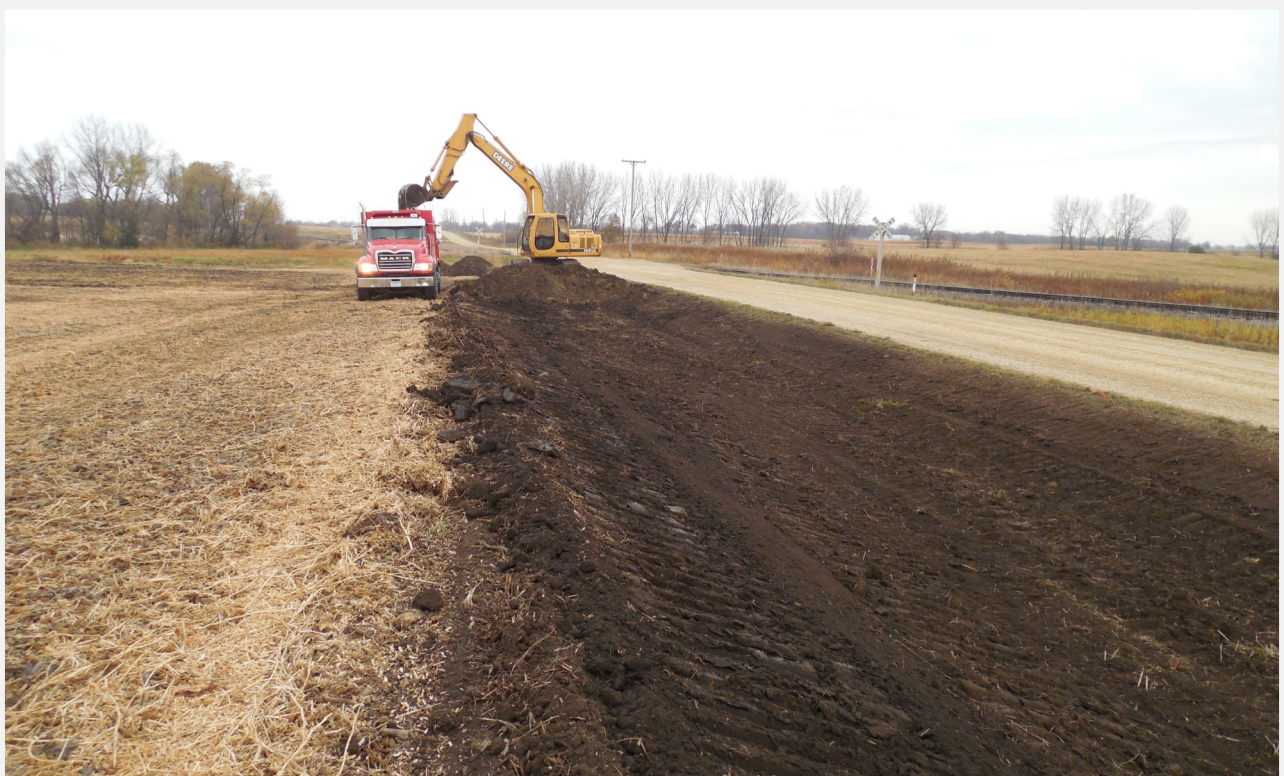
Ditch re-shaping on central area of Eveleth Avenue
