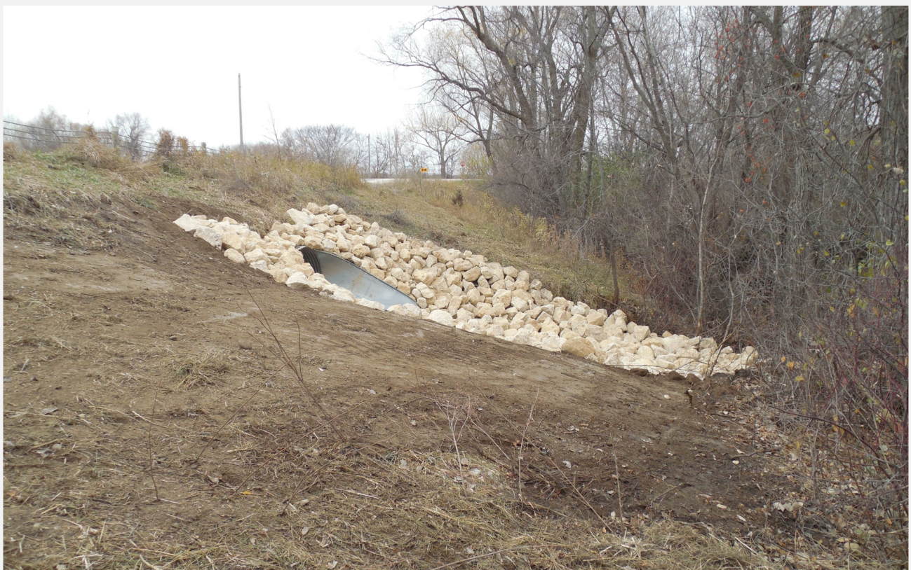
Repaired culvert and erosion control project on the East side of the northend of Holyoke Avenue.
