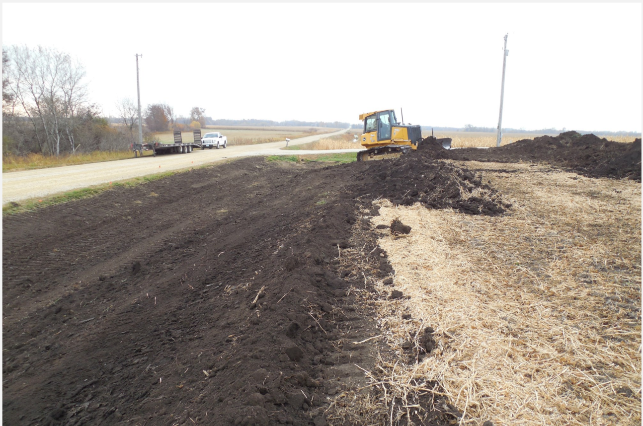
Ditch shaping on the West side of Eveleth Avenue
