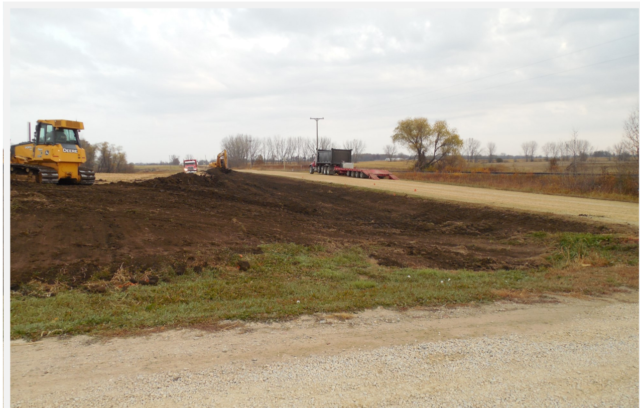
Ditch shaping on the West side of Eveleth Avenue
