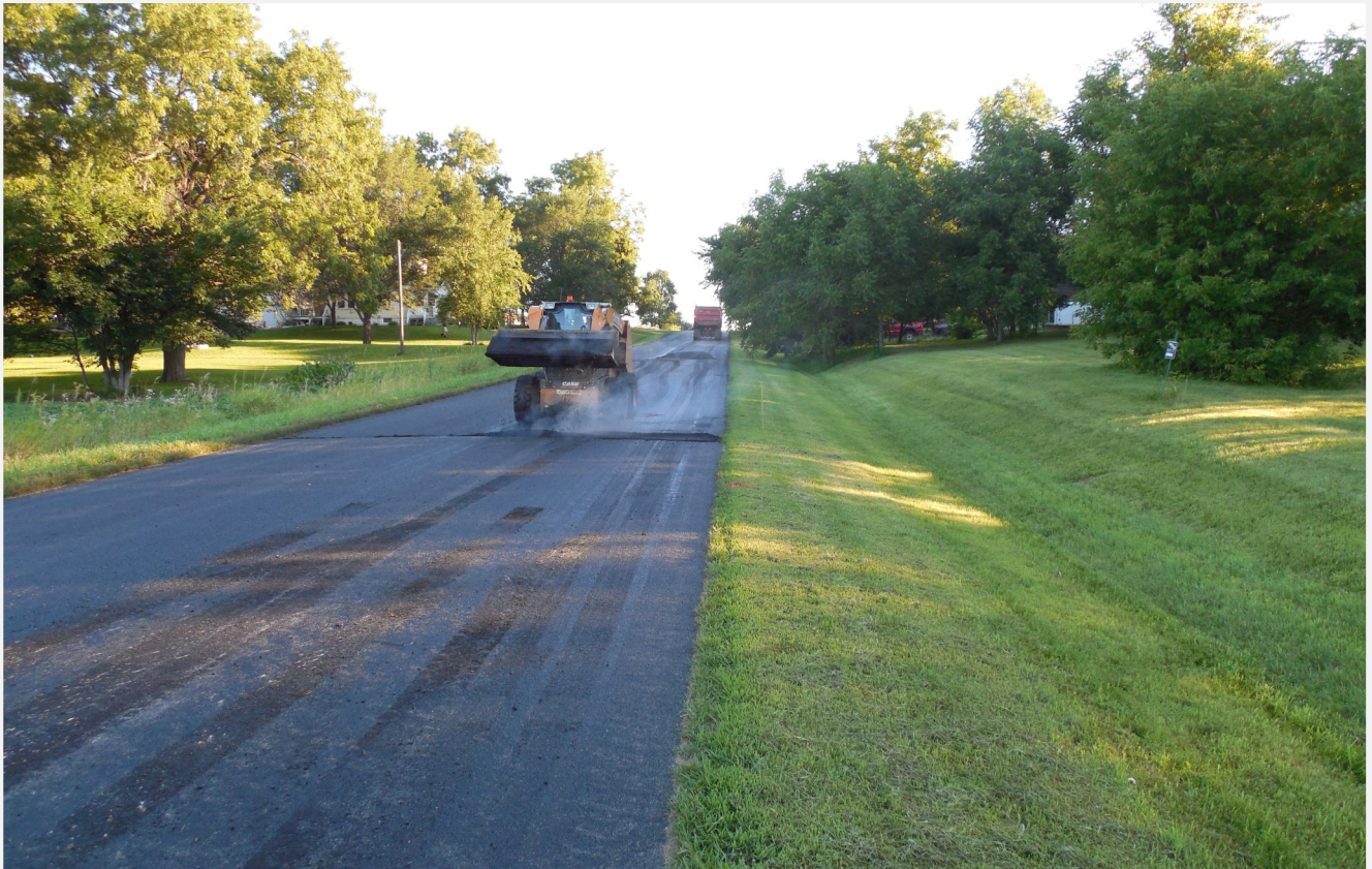
Repairing cracks and “tight grading” Dresden Avenue before paving.
