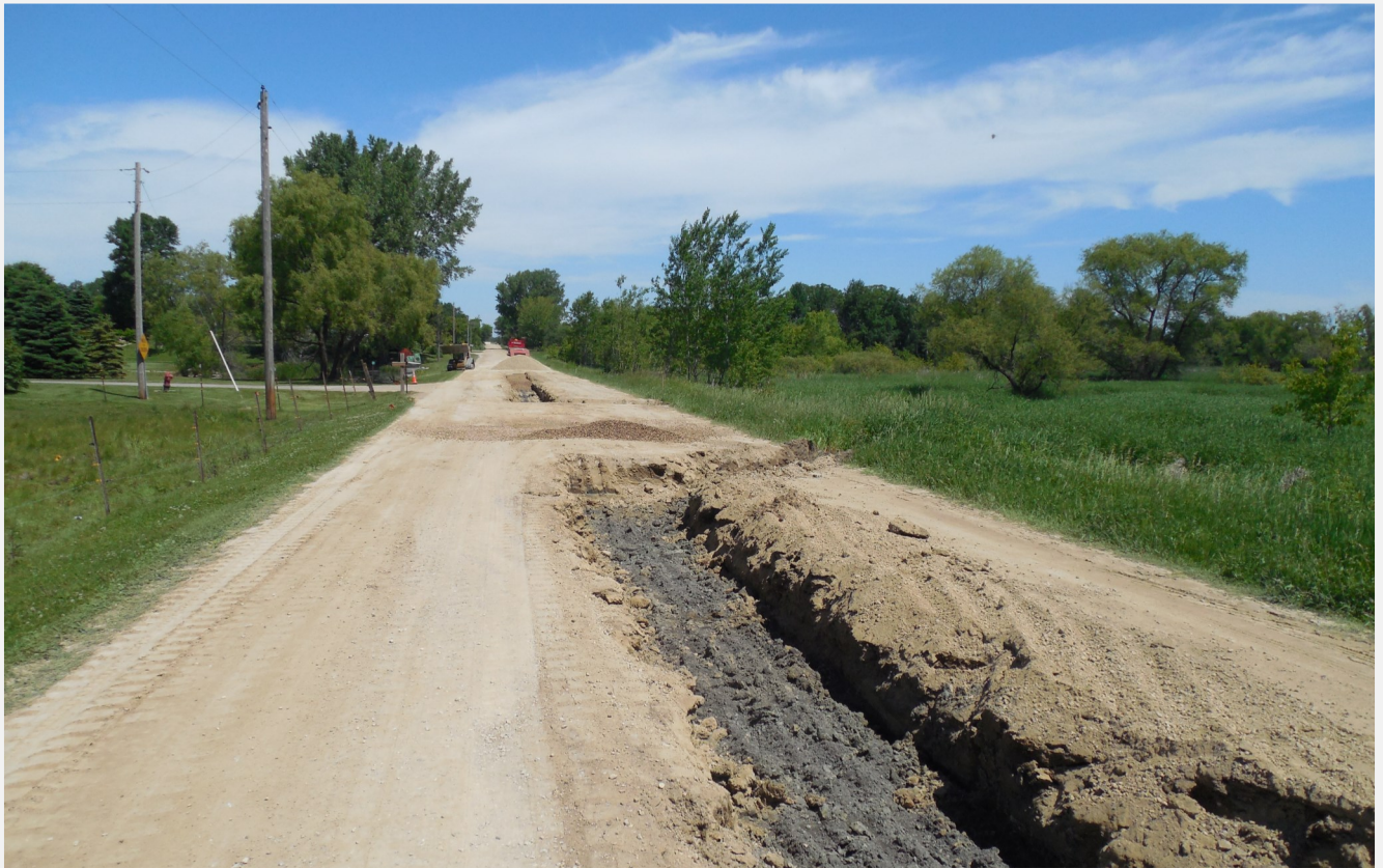
Frost boil repairs. Mid-section, Jamaica Avenue.
