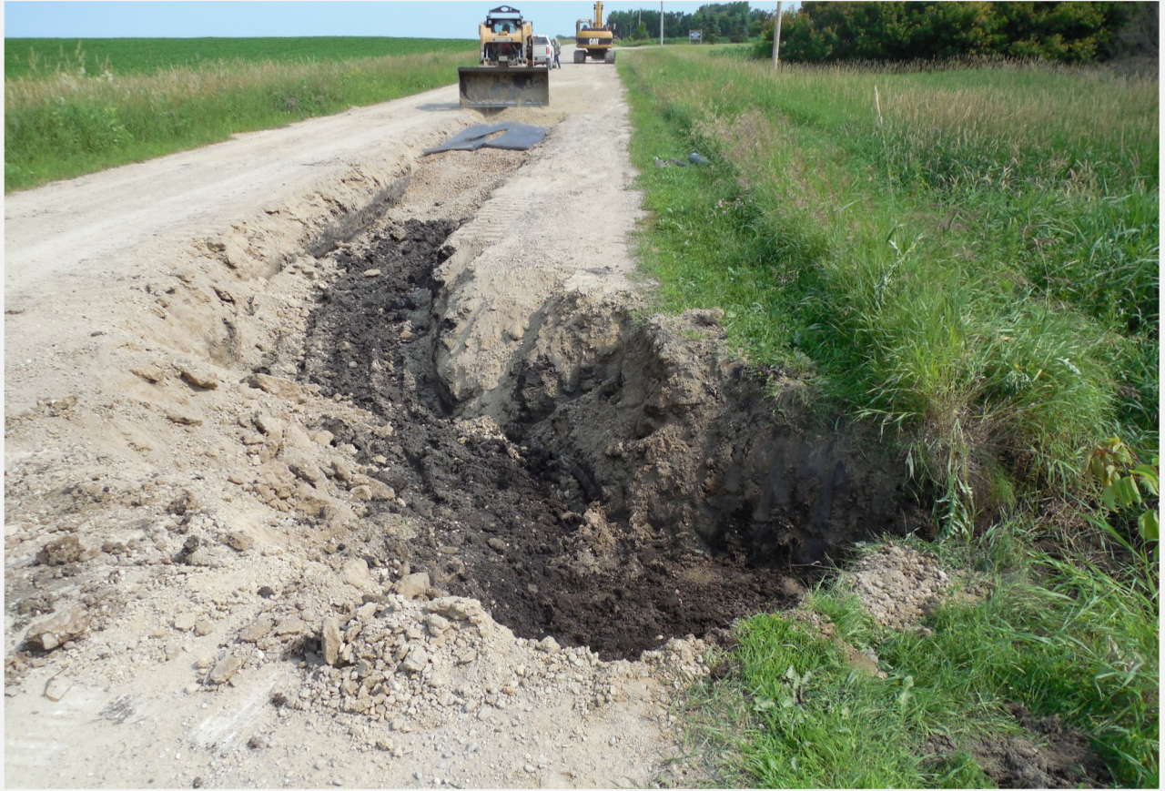
Frost boil repairs. South of Town Hall on Guam Avenue.
