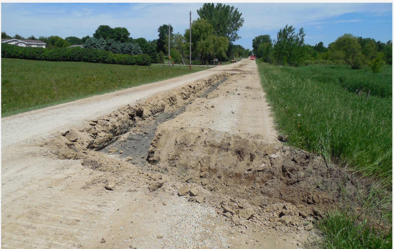
Frost boil repairs. East side, middle area of Jamaica Avenue
