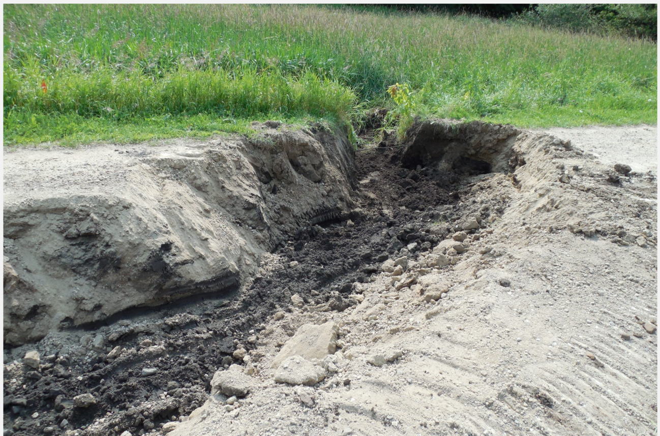
Repairing frost boils. South end of Guam Avenue.
