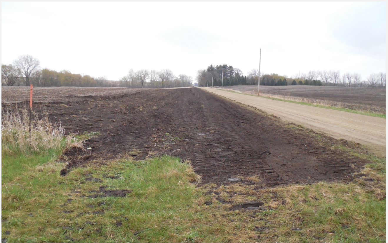
Cleaned and reshaped ditch. North side of 285th Street West
