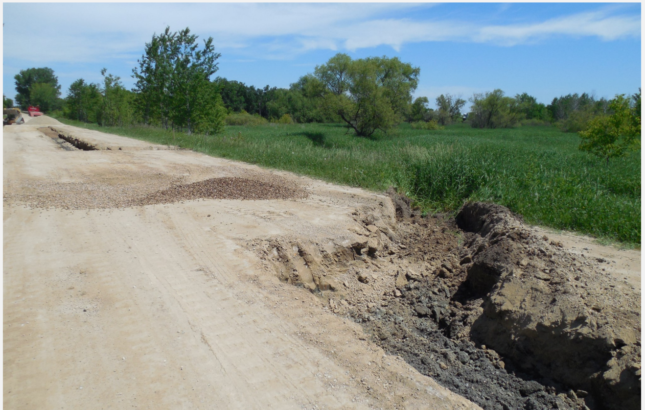
Frost boil repairs on Jamaica Avenue.
