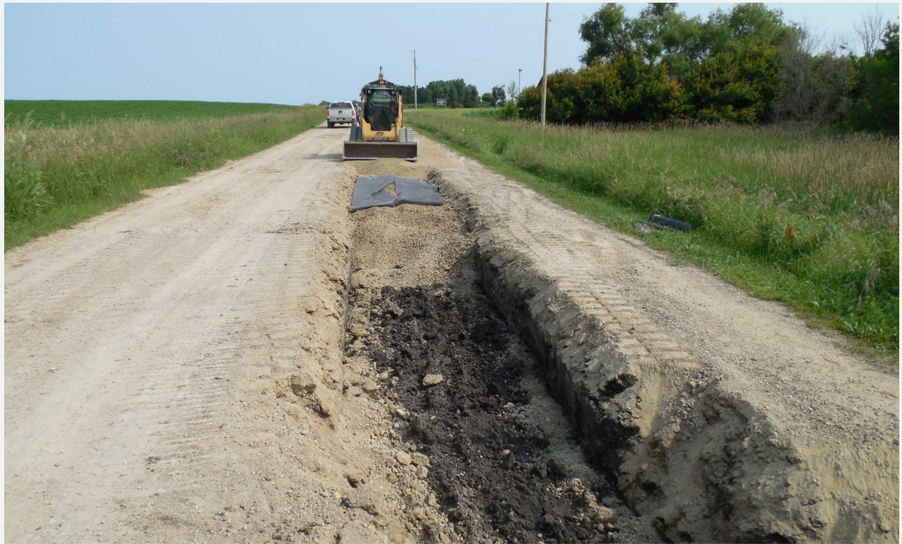
Repairing frost boils south of Town Hall on Guam Avenue.
