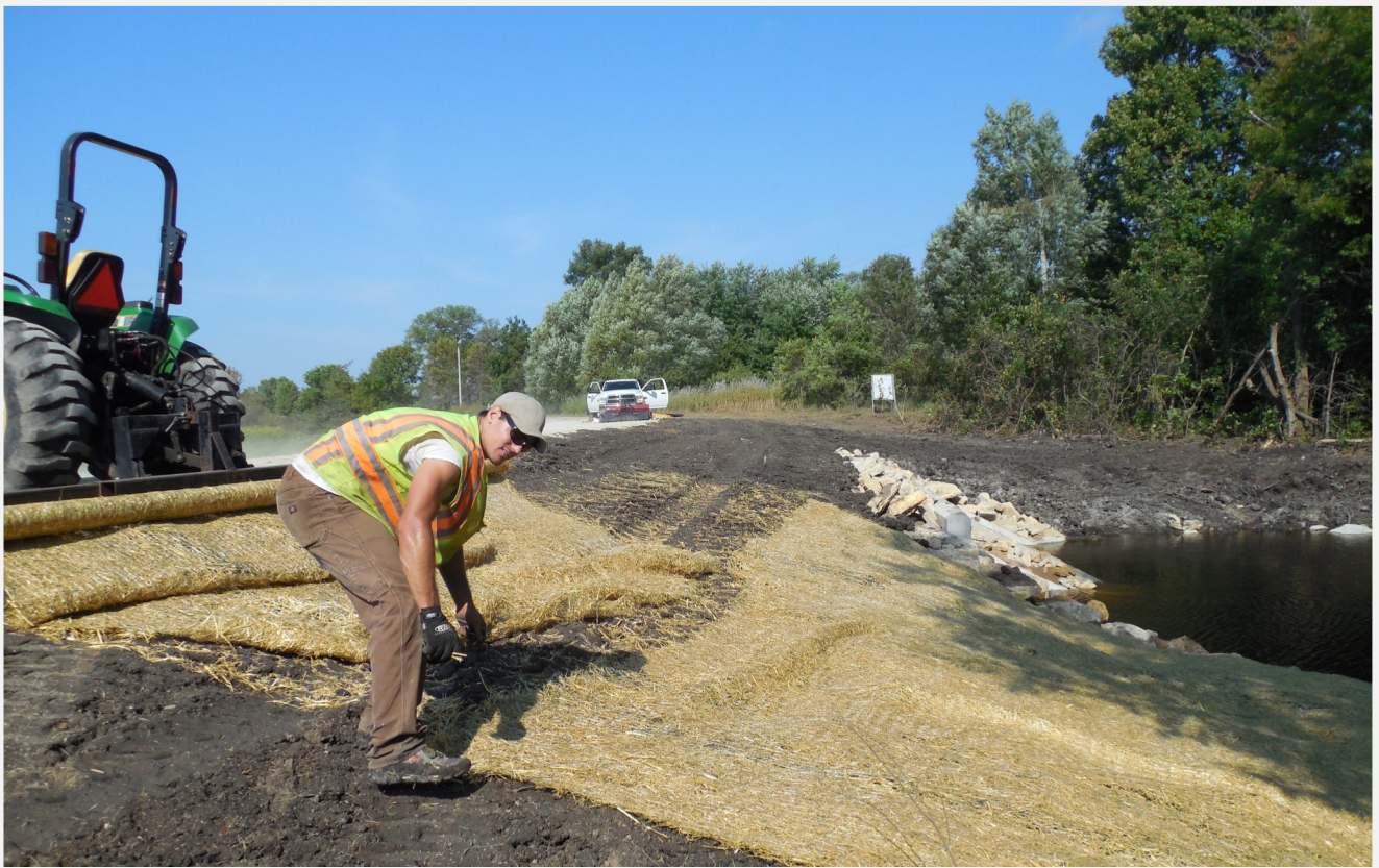
Erosion control work on bridge site on Dakota County #90.
